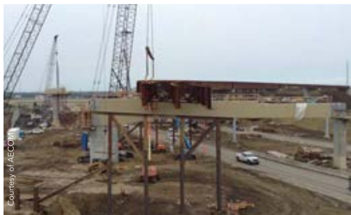
FIGURE 4: Bridge 23.3 Girder Erection (Pier 5 to Abutment 1)
