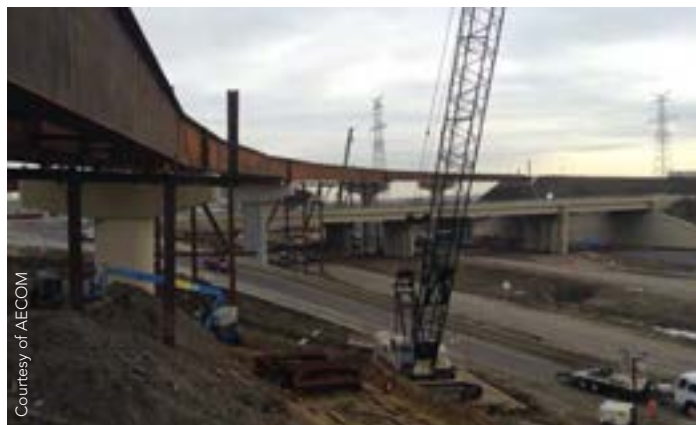
FIGURE 6: Bridge 23.5 Girder Erection Completed (Pier 4 – Abutment 1)
