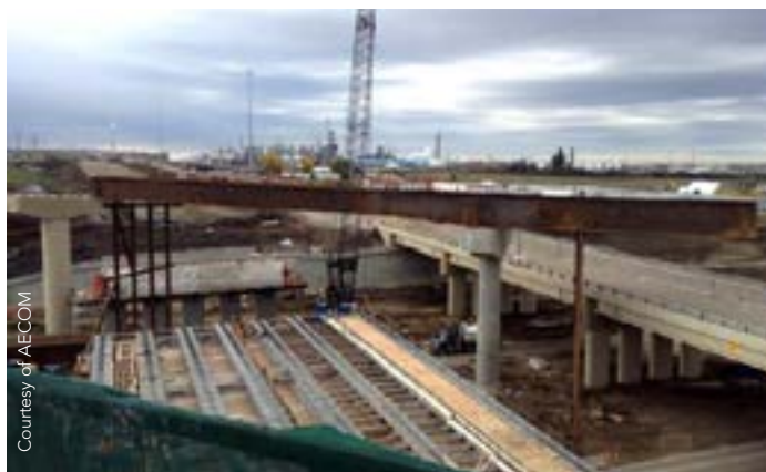
FIGURE 5: Bridge 23.5 Girder Erection (Pier 1 to Pier 2)
