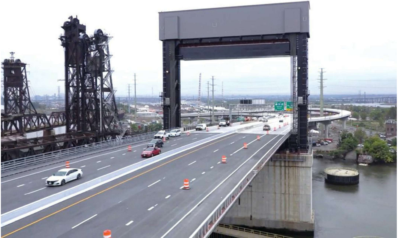
The new Wittpenn Bridge is New Jersey's first orthotropic bridge and an integral component of the state's Portway Corridor project. Courtesy of CCA Civil »
