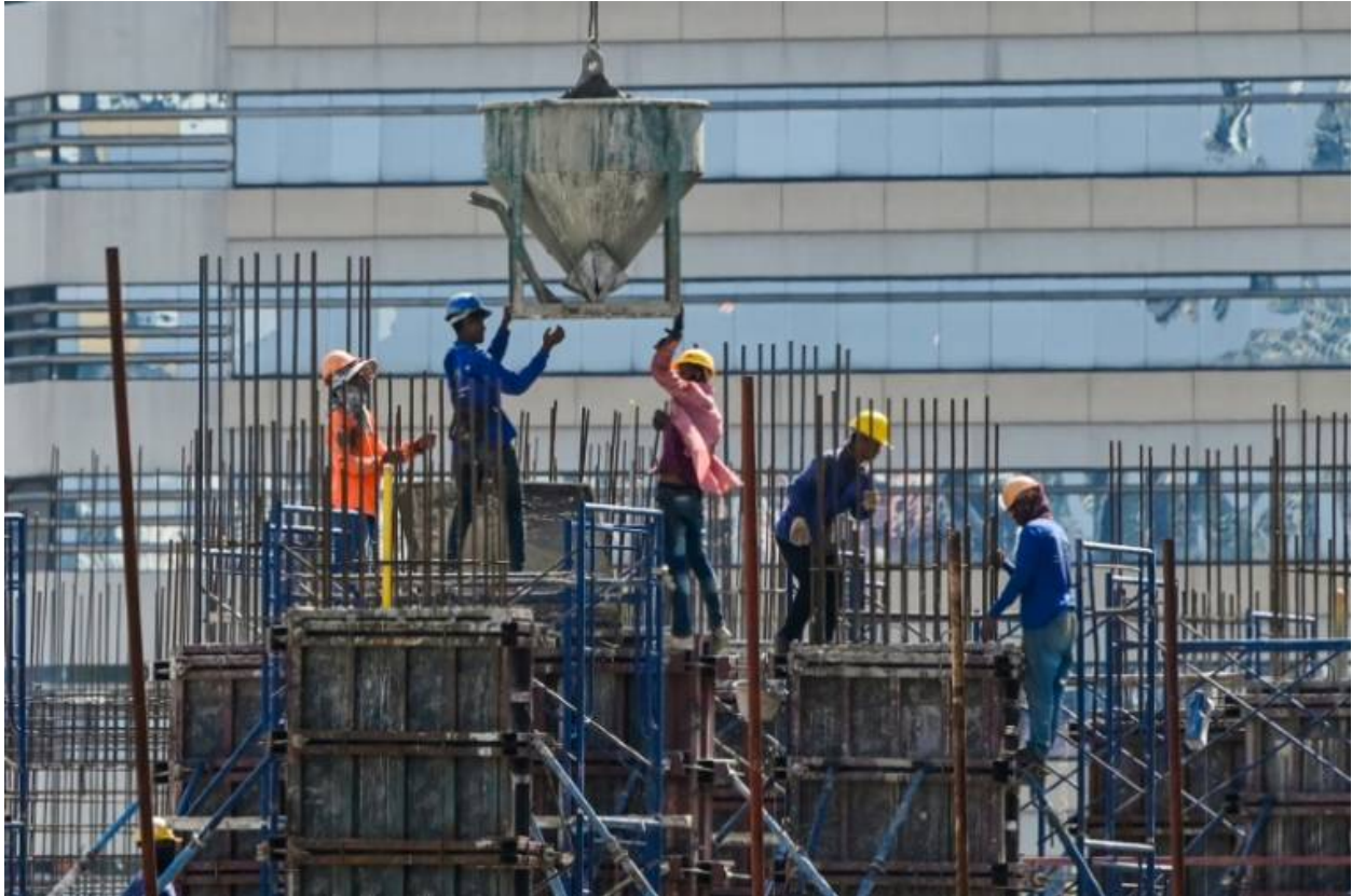
A building under construction in Bangkok, May 16, 2020 ( AFP / Romeo GACAD )
