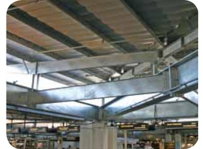
Hot-dip galvanized structural beams.
