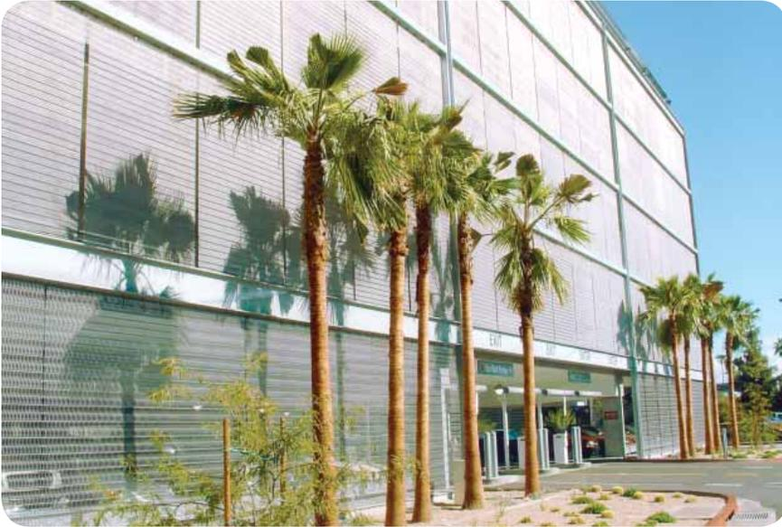
The expansion of Arizona State University recently included the construction of a large, five-story parking facility. Hot-dip galvanized steel was used in this parking garage for its aesthetic appeal and also to protect the automobiles from UV rays and other corrosive elements in Arizona. The parking structure contains many different HDG pieces, including the parking canopy, columns and beams for the skin structure, crash barrier, and guard rails totaling 150 tons (135 metric tons) of steel.
