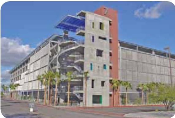
is used to help provide shade and protection from the elements for the parked vehicles. The galvanizer also suggested bolting the frame together in lieu of welding to minimize the size of the pieces that were galvanized, eliminating unnecessary progressive dipping.
