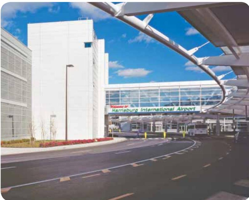
The hybrid structural system, featuring hot-dip galvanized steel columns and beams, in combination with precast double tees, gives the facility a visual openness and a compositional synergy with the mostly-transparent envelope and metal cladding of the new terminal. Galvanizing—functional, versatile, and aesthetically appealing!
