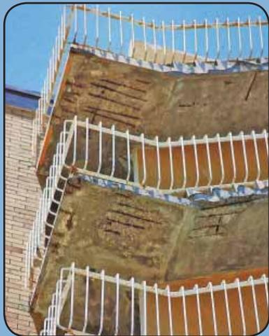
The primary cause of the deterioration is corrosion of bare steel reinforcement. Unless protected by a coating such as zinc, applied in the hot-dip galvanizing process, bare steel will corrode. Because rust occupies a volume 4 to 6 times greater than the original steel's volume, the concrete will inevitably crack, spall, and need replacement.
