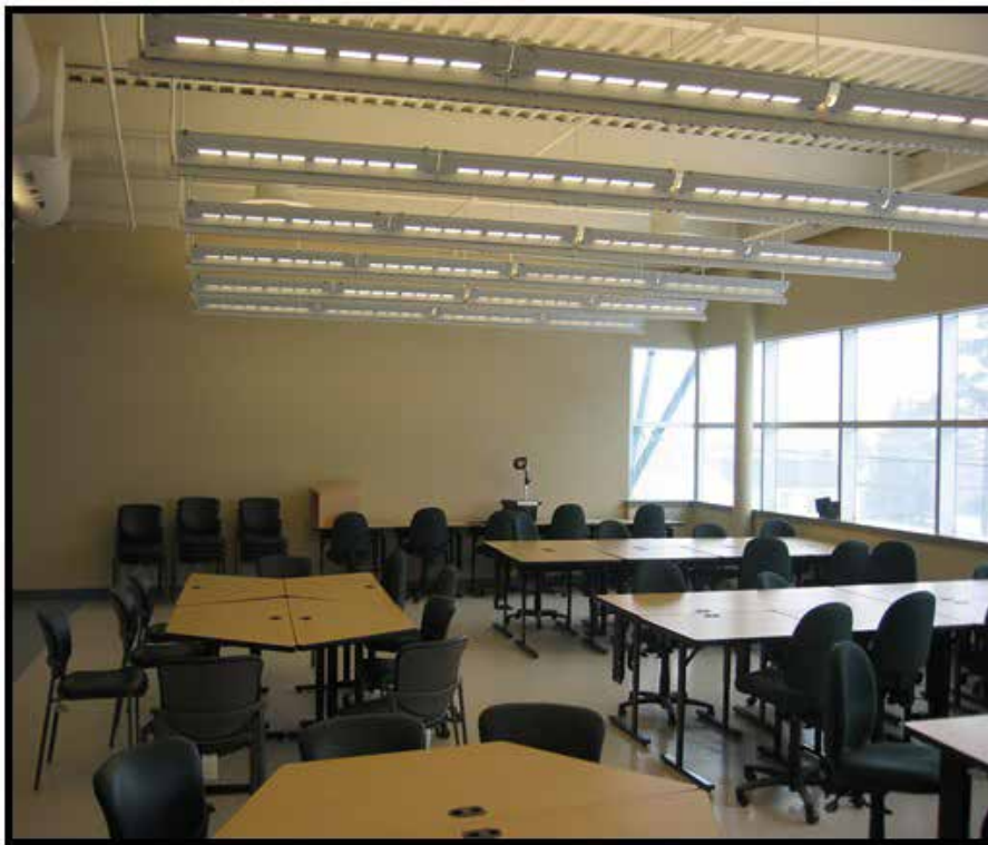
Unprotected exposed steel in floor-ceiling assembly in a classroom at the Nova Scotia Community College and Citadel High School.
