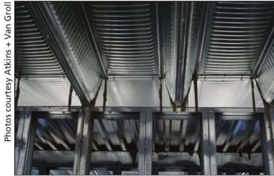
This image shows a deep composite deck on LSF. In deep deck, scallops form a concrete beam over the top of the load bearing wall, which helps to disperse the load.
