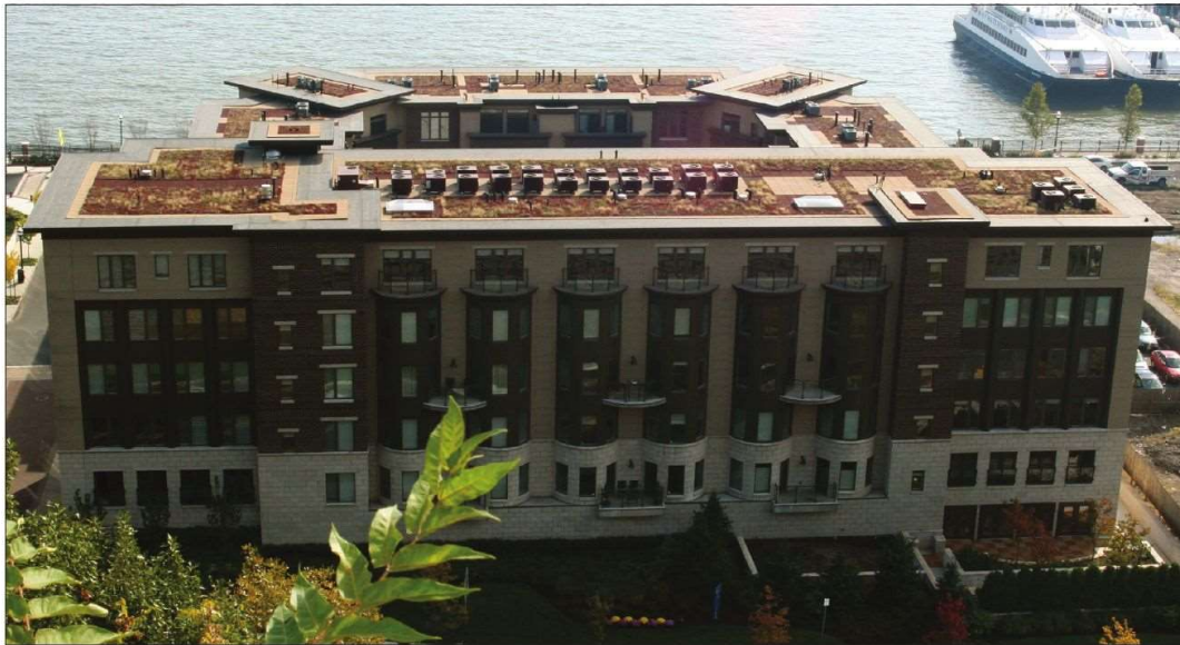
Henley on the Hudson, high-end condominiums in Weehawken, New Jersey, use deep deck and LSF. Specialty curved panels are prefabricated and include insulation and exterior finish.
