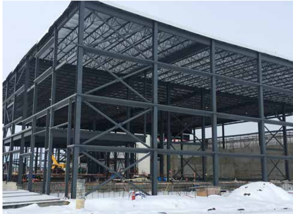
FIGURE 1 A four-tiered concentrically braced frame in an industrial building.
