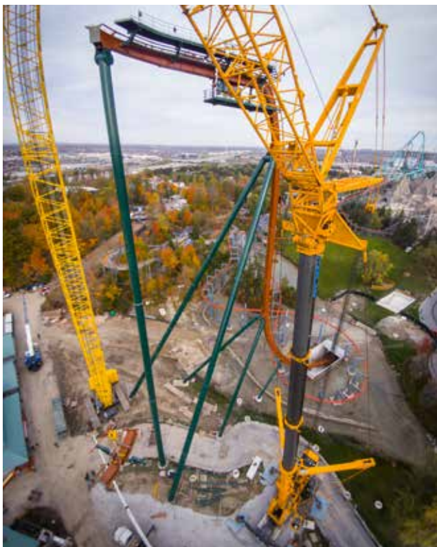
A bird's eye view of two cranes lifting track elements to record-breaking heights.
