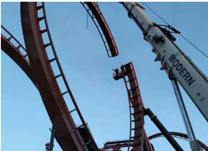
Ironworkers guide the last track element into place for a 360-degree loop.
