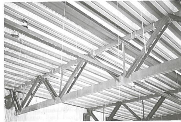
FIGURE 4.13 Trusses with HSS chords and angle web members
