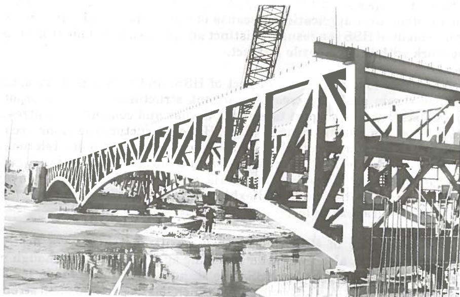
(b) HSS bridge under construction
