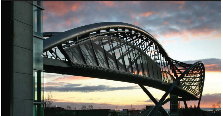
Helix Bridge, Seattle Washington - 36" O.D. x 1.25" wall and 24" O.D. x 1" wall bent to a multiple radius helix
