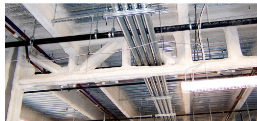
FIGURE 2: Special Truss Moment Frame - Minetta (San Jose) International Airport
