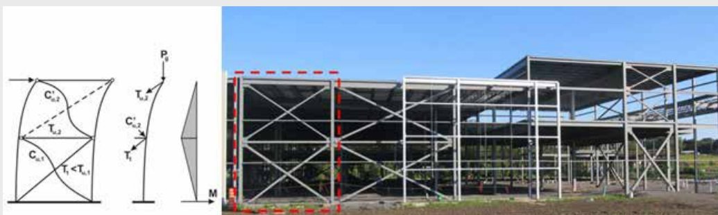
FIGURE 1: Multi-Tiered Braced Frame
