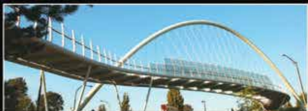
Passerelle Griffiths Drive, Burnaby, C.-B. – 24 po (DE) x 7/8 po (paroi)
