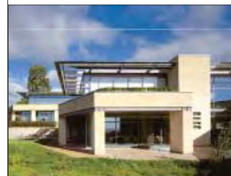
Figure 1: Wessex Water headquarters achieved one of the best environmental ratings for an office building in the UK using a steel frame with precast concrete floors
