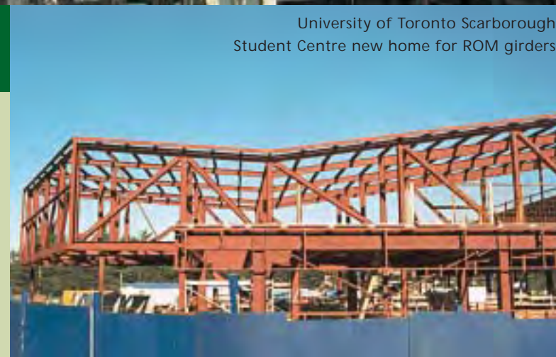
University of Toronto official, for accepting the (donated) steel. This administrative aspect had to be factored into the project scheduling of this reuse. The reused steel amounted to approximately 18 tons of saved steel.
